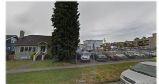
View from South of site along London Street, showing neighbor's house
