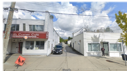
East side of twelfth Street, site on left of lane, neighbor on right of lane
